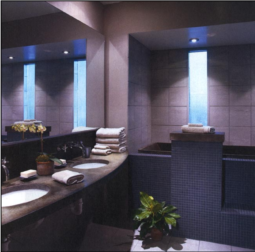
The master bath's double vanity and bathtub are custom concrete castings.
